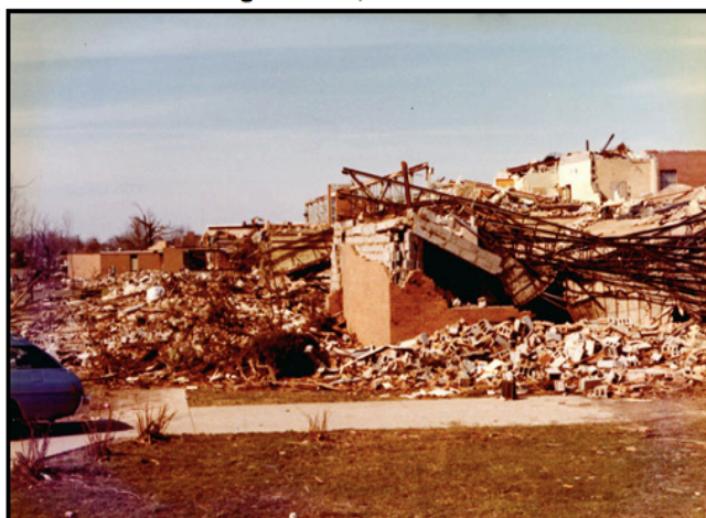
EF5 Tornado Damage - Xenia, Ohio 04/03/1974
