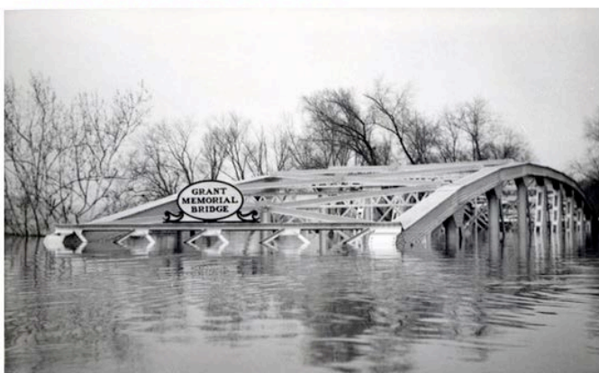
The Grant Memorial Bridge in Point Pleasant.
