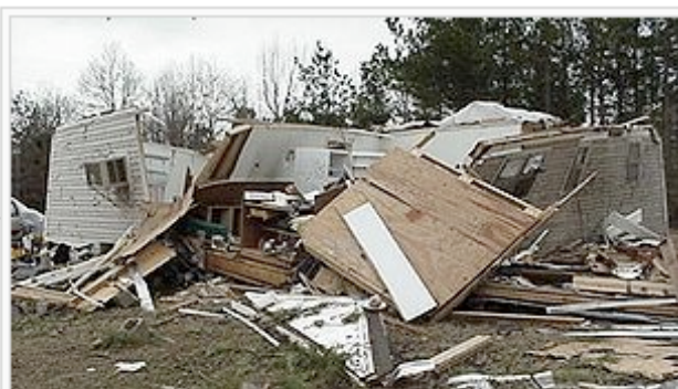
An example of F2 damage. At this intensity, tornadoes have a more significant impact on well-built structures, damaging roofs, collapsing walls, and generating large amounts of flying debris. This wood-frame home was unroofed, with many outer walls collapsed or destroyed.
