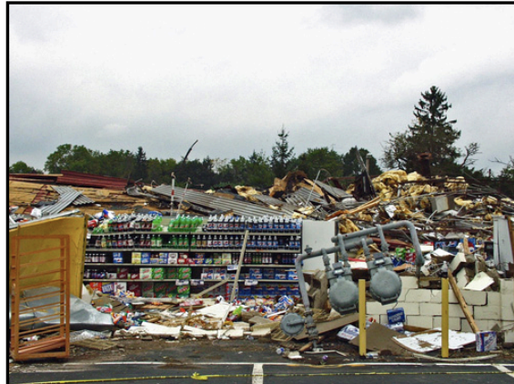
EF3 Tornado Damage - Xenia, Ohio 09/20/2000
