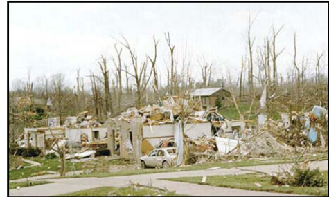
EF4 Tornado Damage - Blue Ash, Ohio 04/09/1999
